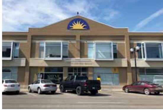
The Dr. Foster James Penny building in downtown Lethbridge provides a central space for the University of Lethbridge to engage with the broader community.
